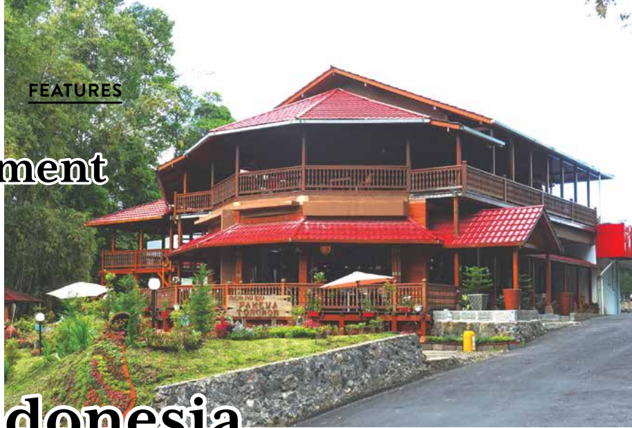
Two Michi-no-Eki facilities have been opened in Indonesia thus far. This one shows Michi-no-Eki Pakewa.
